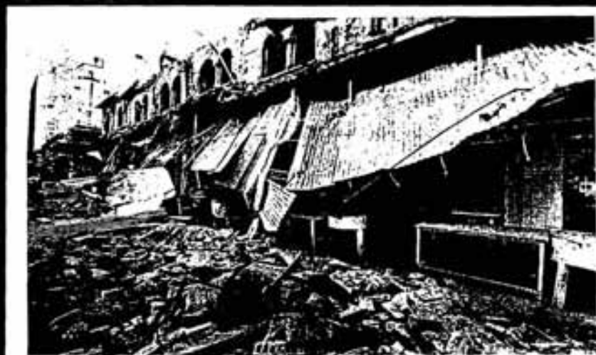
Fig. 17 The Central Market in Thessaloniki after the main shock. The buildings were erected in the last quarter of nineteenth century (from a local newspaper).
